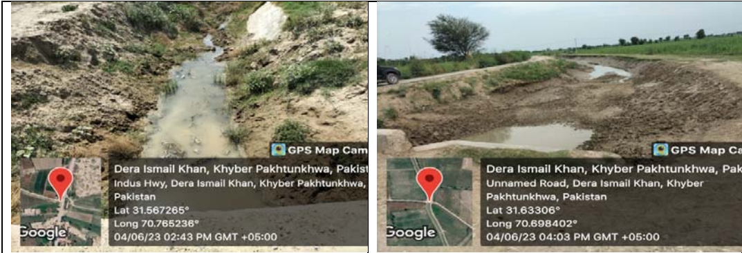
Rehabilitation of damaged / washed away Drains Section of Bilot Creek Drain
