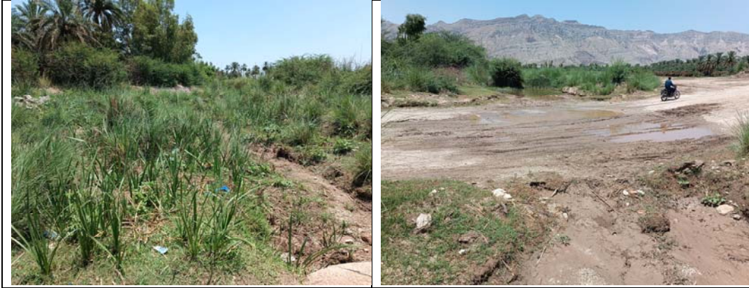
Rehabilitation of Katgarh Branch Drain No. 03
