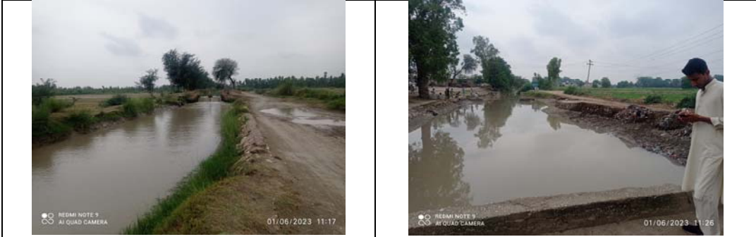
Rehabilitation of damaged/washed away Canal Section of Paharpur disty
