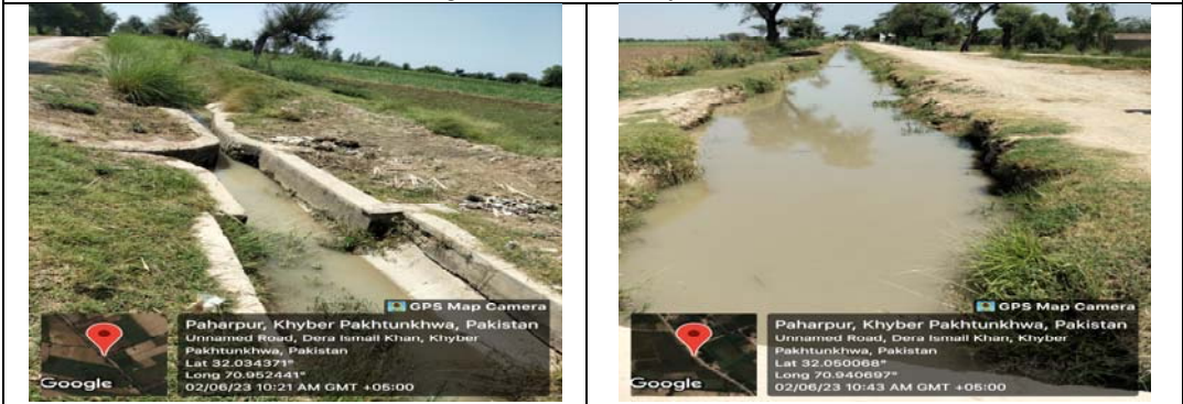
Rehabilitation of damaged/washed away Canal Section of Civil Minor
