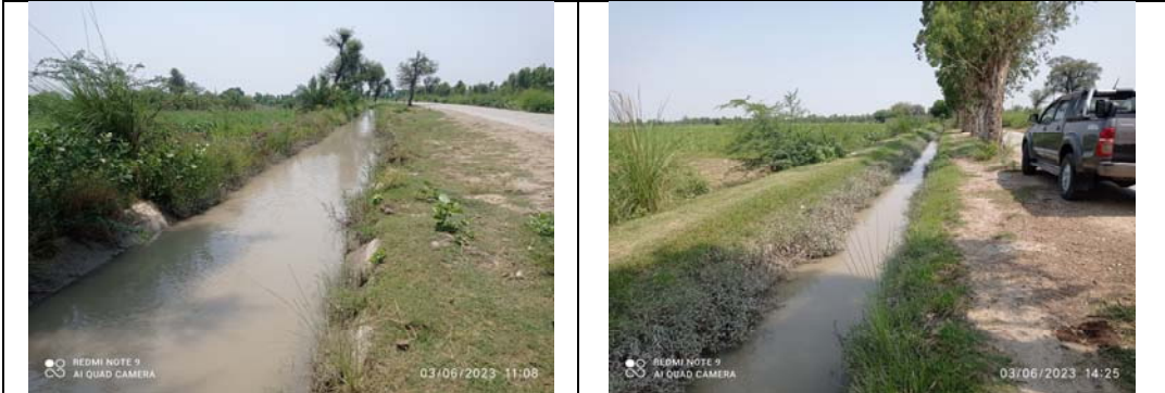
Rehabilitation of damaged/washed away Canal Section of Ketch Minor
