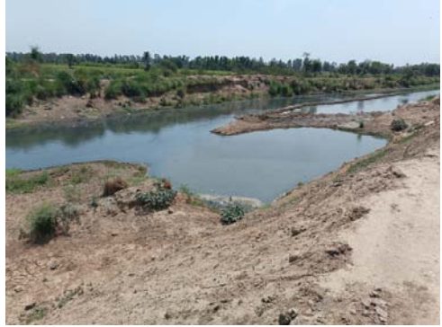
Rehabilitation of damaged / washed away Drains Section of Main Drain
