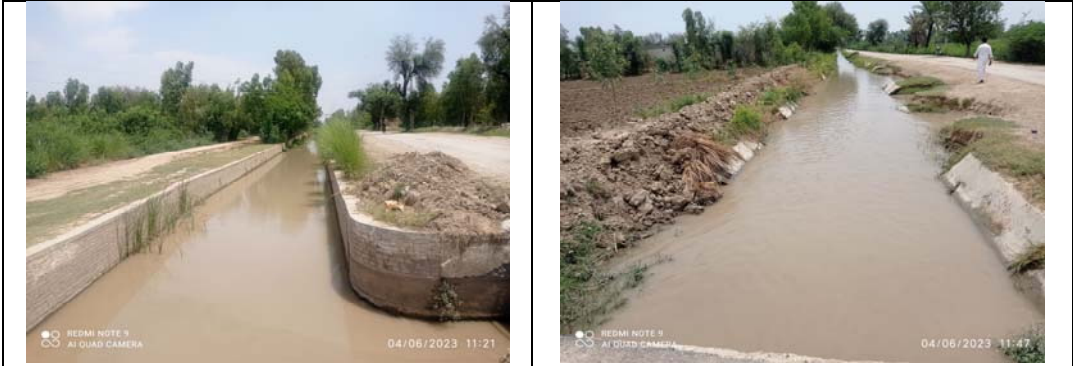
Rehabilitation of damaged/washed away Canal Section of Shah Kot Minor
