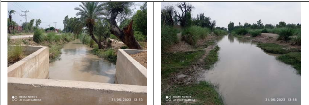
Rehabilitation of damaged/washed away Canal Section of Shah Kot Feeder
