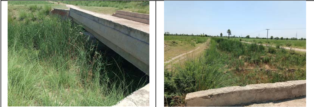
Rehabilitation of Katgarh Branch Drain No. 04
