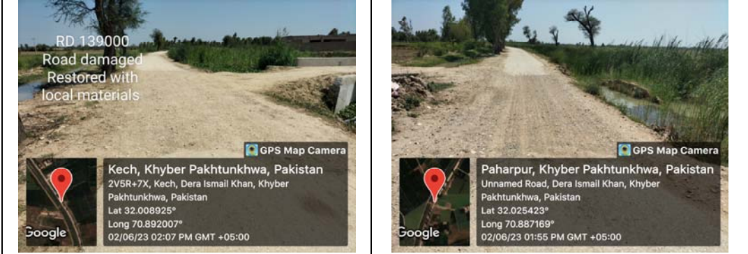
Rehabilitation of damaged/washed away Canal Section of Old Paharpur canal (RD. 130000-160000)
